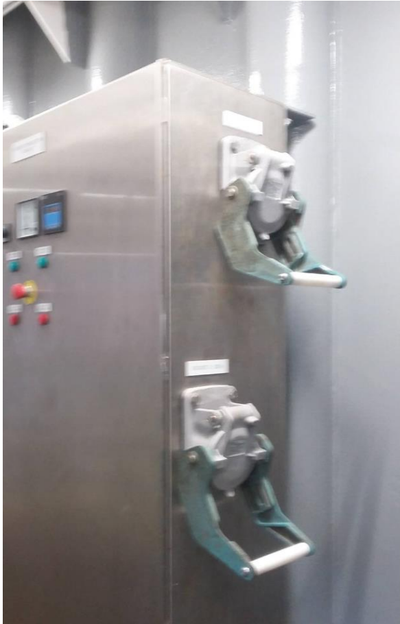
Cavotec connection Olympic Energy
